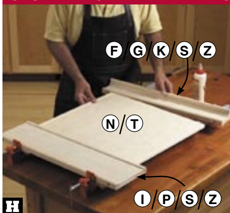
H Squeeze glue into the end lower rail (I/P/S/Z) and end upper rail (F/G/K/S/Z) grooves, and clamp the panel (N/T) in place.
